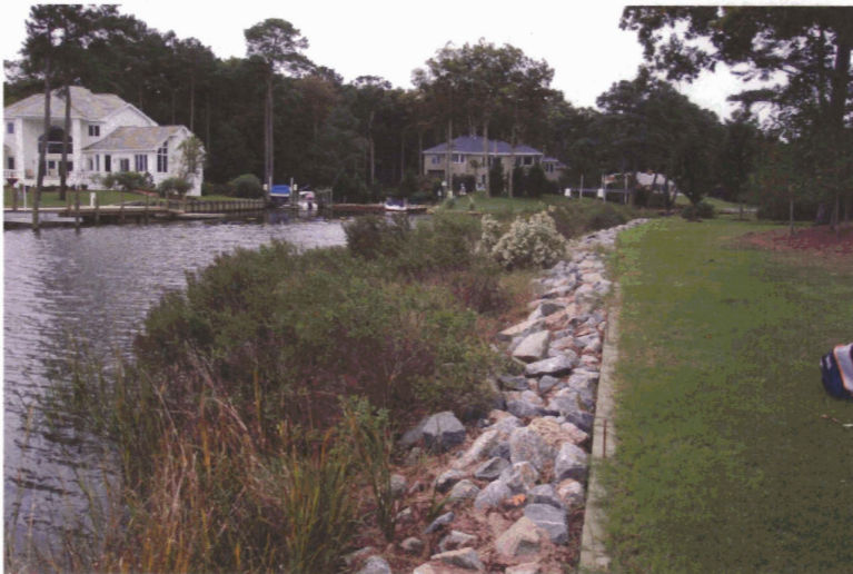
Figure 18 96-V0527 Olmstead Site
